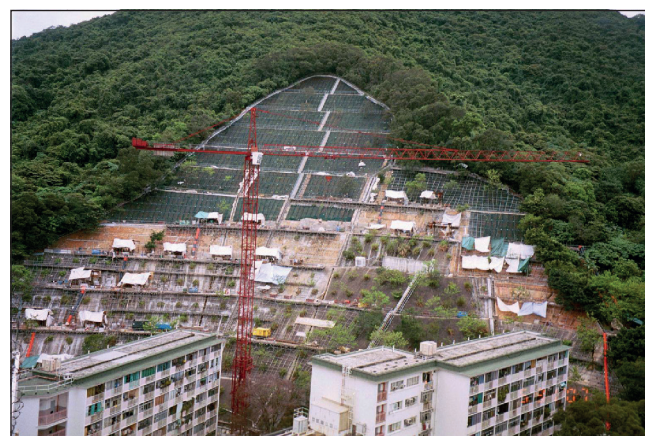
Figure 5. Construction of hand-dug caissons at Sai Wan Estate, Hong Kong
