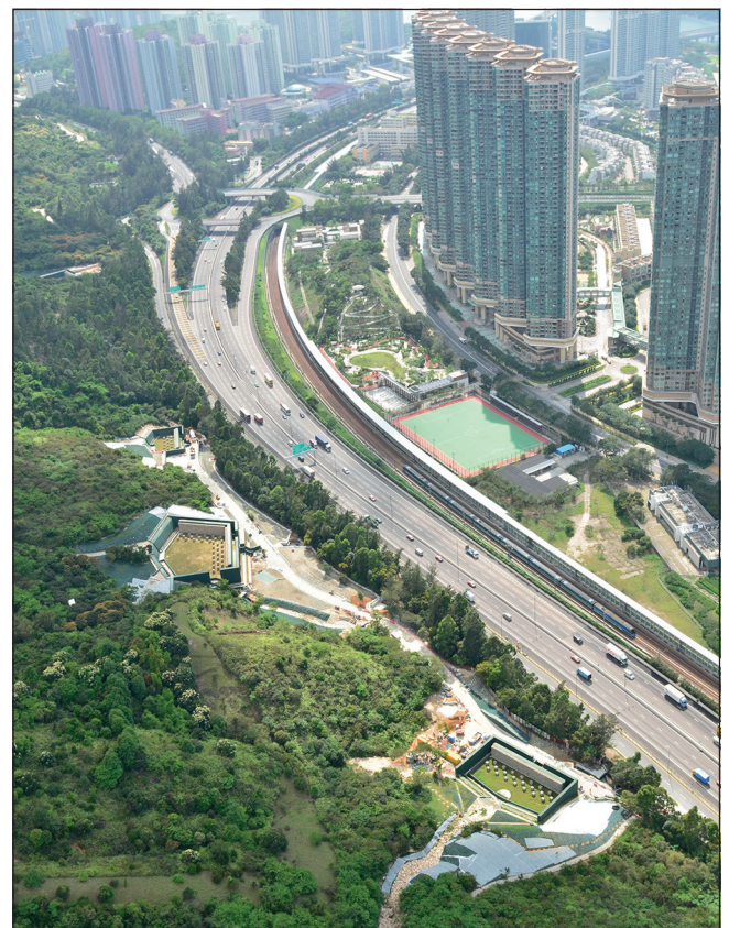
Figure 9. Concrete check dams at the toe of natural hillside
