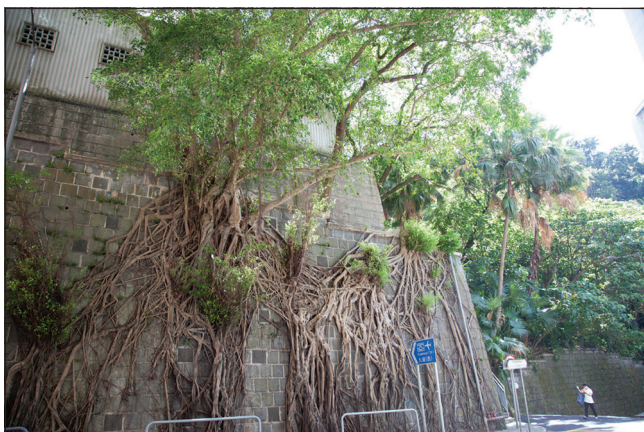
Figure 7. Old masonry wall upgraded with the use of soil nails
