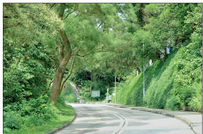
Figure 8. Landscape treatment on an upgraded roadside cut slope
