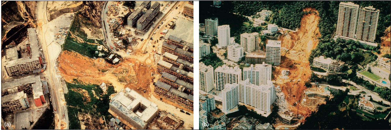
Figure 1. Disastrous landslides on 18 June 1972 in Hong Kong: (a) Sau Mau Ping (71 fatalities); (b) Po Shan (67 fatalities). From 1977 to 2010 approximately HK$19 billion (about £1.9 billion) was spent on landslide prevention measures
